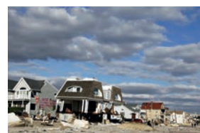
Homes were damaged.
